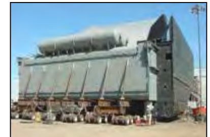
Removable Spillway Weir
